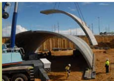
The finished arch underpass is six metres high with a span of 18 metres
