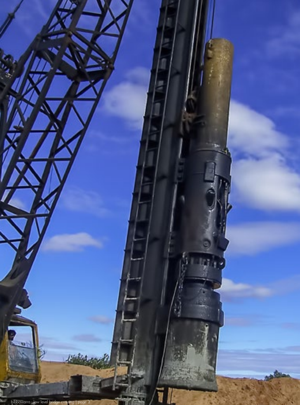
bibbawarra - low level bridge crossing | page 3
