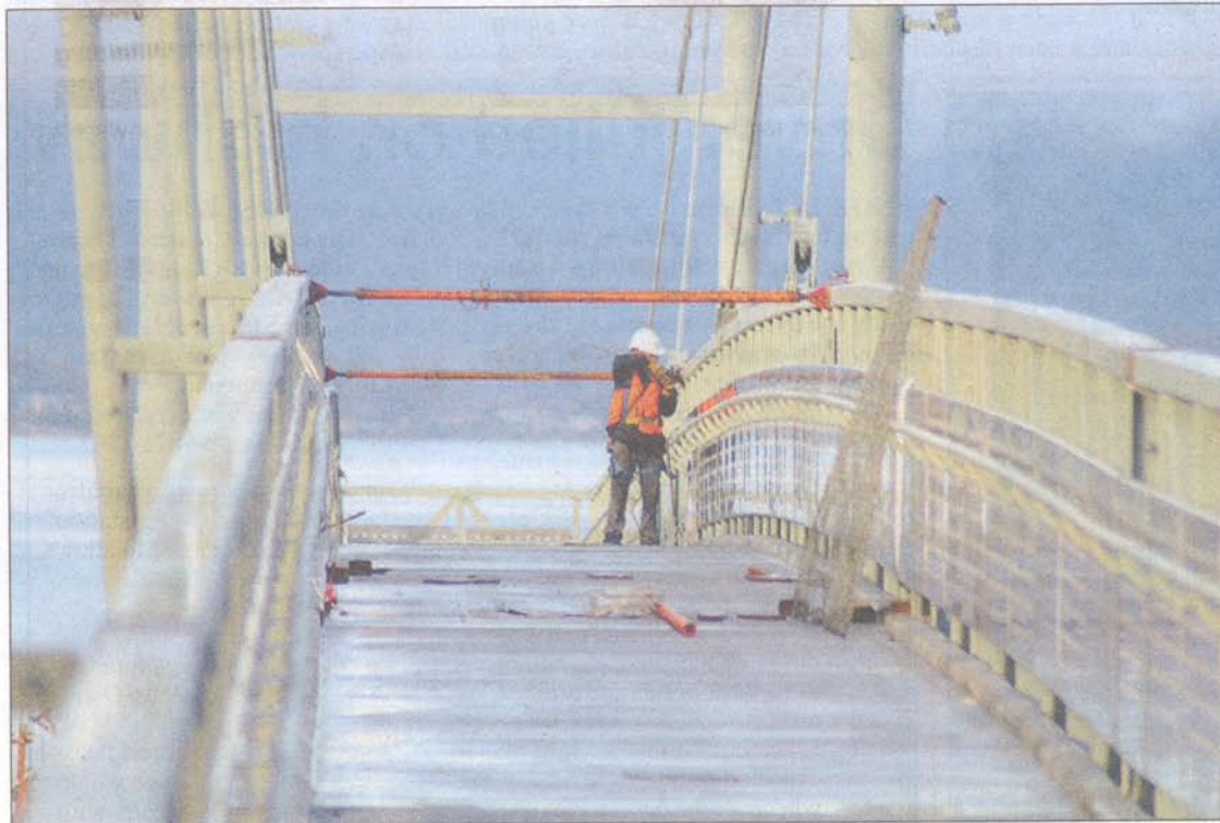
Work being completed on the final section of the pedestrian footbridge.
