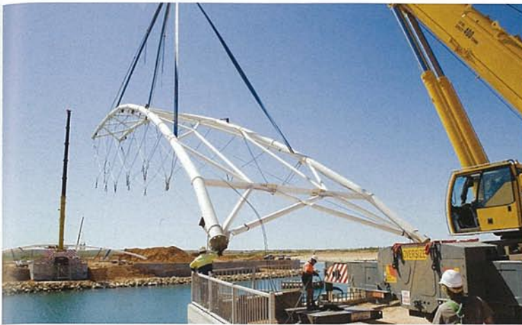
Left and right: Construction photographs showing the arch being installed over the canal
